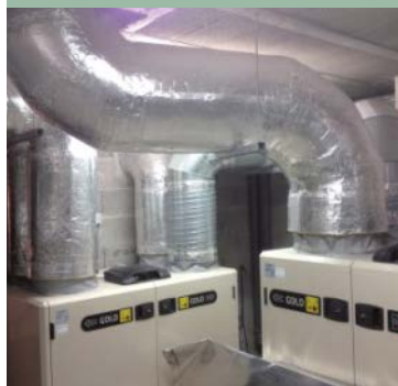
2 centrales de ventilation double flux Abibois ©
