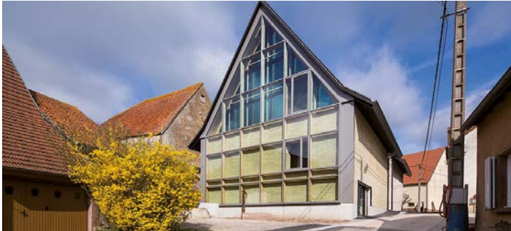
Luc Boegly, Nunc Architectes ©
